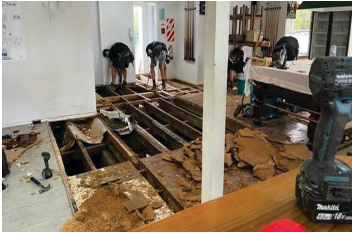
Wardy Construction team who worked like 'Trojans'
